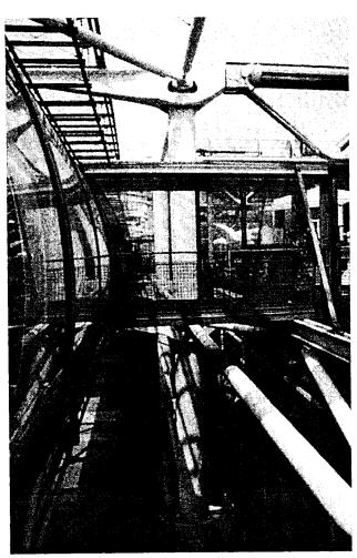
Fig. 5. Centre Pompidou, top level. Circulation elements around a gerberette member.
